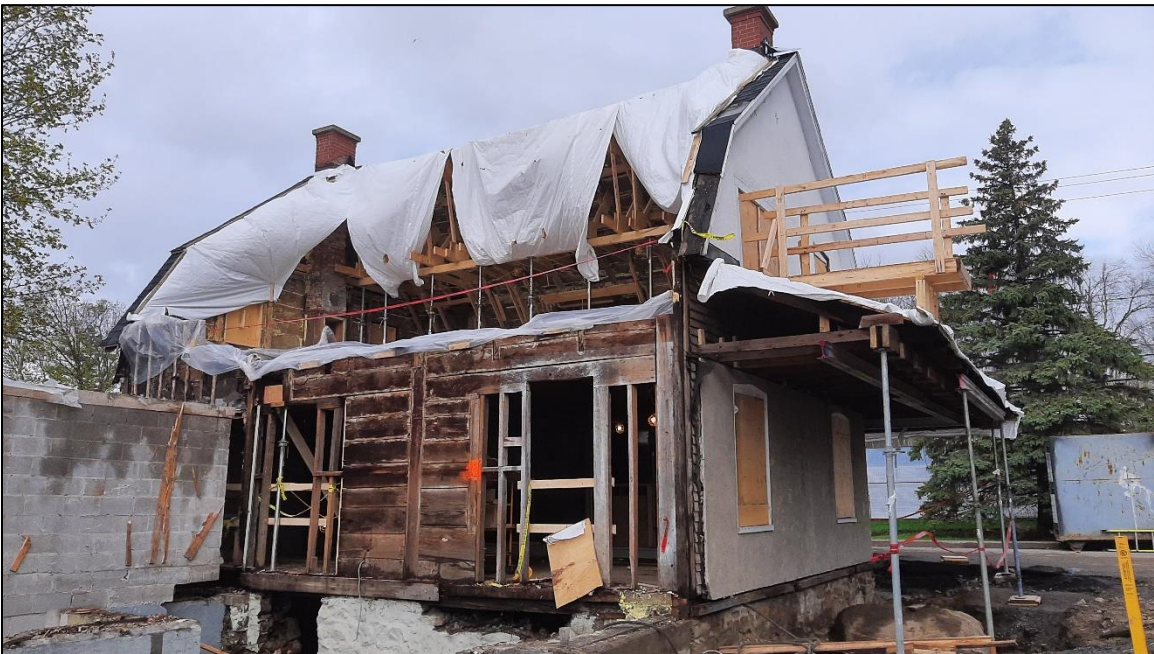
Photo 17. Rear view of the current building, during the refurbishment works. It shows the structure made of wooden planks (BiFI-18-23-N2-43).
