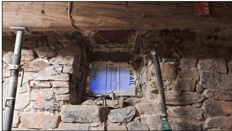
Photo 9. Detail of the interior facing of the west wall of the building. Here, one can see one of the western red cedar beams as well as the old opening leading outside, now sealed. View towards the west. (BiFI-18-23-N2-25).
