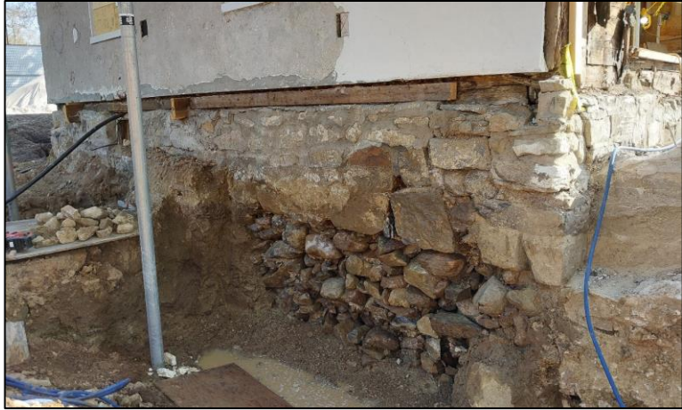
Photo 20. Overview of the exterior facing of the west foundation wall of the City Hall building. The distinction between the above-ground portions and the underpinning (unjoined) is very clear. View towards the northeast (BiFI-18-23-
